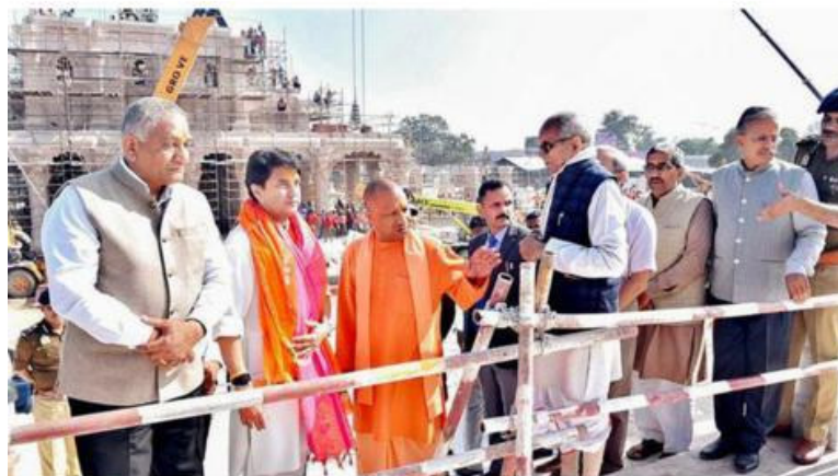
Taking stock: Chief Minister Yogi Adityanath, and Union Ministers Jyotiraditya Scindia and V.K. Singh inspect the construction of the Ram Temple ahead of its inauguration, in Ayodhya on Saturday. | Photo
