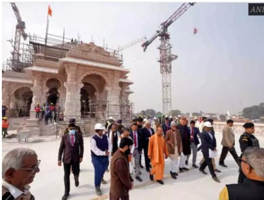
Construction work at Ayodhya
