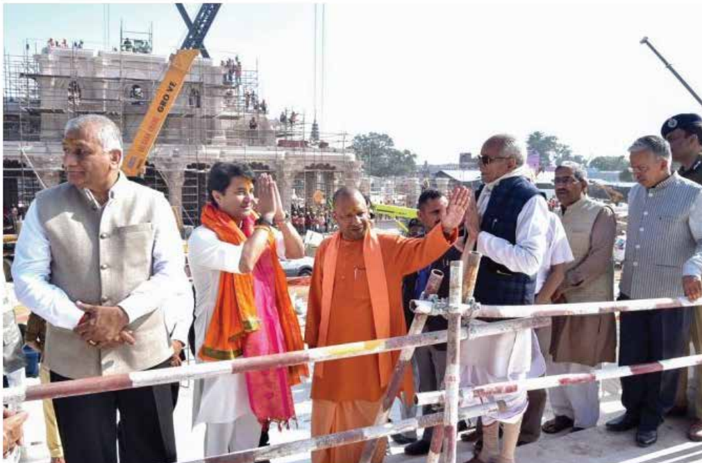
IMAGE: Union Civil Aviation Minister Jyotiraditya Scindia (second from left) with UP Chief Minister Yogi Adityanath (second from right) and Union Minister of State for Road Transport and Highways General (Retd) VK Singh (left) visit Ram Mandir construction site, in Ayodhya, December 2, 2023. Photograph: ANI Photo
