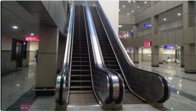
The revamped railway station is among several projects of the Centre under execution in Ayodhya. (Ravinder Singh/ HT)
